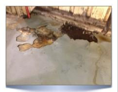
Poor preparation and bond of previous coating systems where also visible throughout the facility. CPI Industrials preparation included the removal of these loose and failing coatings down to the concrete to insure the bond of the new urethane mortar application.
