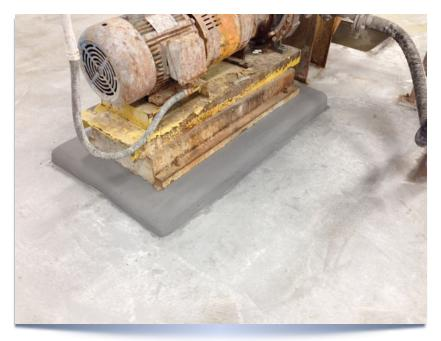
CPI Industrial rebuilt the pump pad and the inside of the sump.
