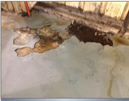
Poor preparation and bond of previous coating systems were also visible throughout the facility. CPI Industrials preparation included the removal of these loose and failing coatings down to the concrete to ensure the bond of the new urethane mortar application.
