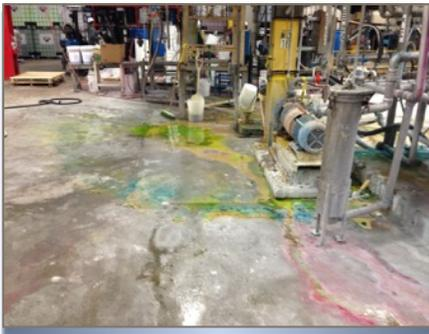
CPI's experience and invested commitment to preparation was invaluable in a project like this. The damaged concrete and old coatings had to be removed to help ensure a good substrate for the new flooring system to bond to. This will help the new flooring system provide years of service.
