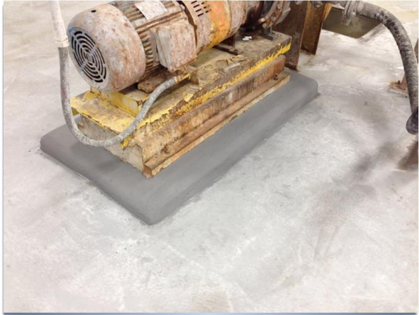
CPI Industrial rebuilt the pump pad and the inside of the sump.
